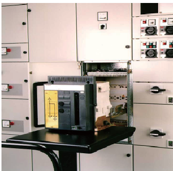
Circuit Breaker Cabinet 6
