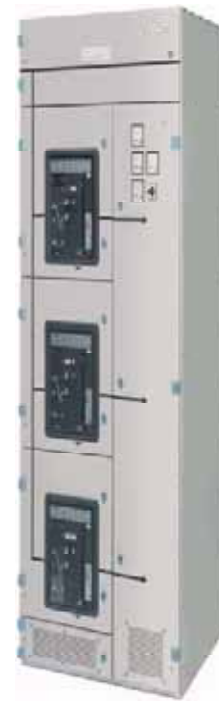
Circuit Breaker Maintain Position
