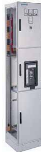
Circuit Breaker Cabinet 2
