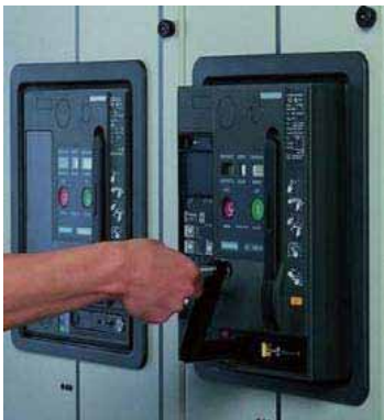
CIRCUIT Breaker DOOR Closed PIX
