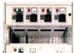
withdrawable module 1, 2, + withdrawable cabinet empty
