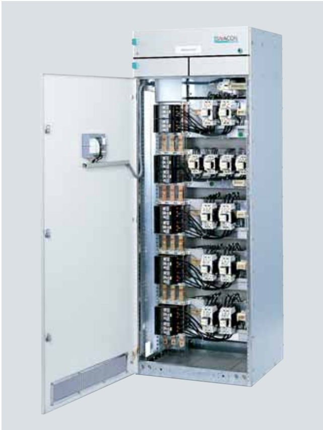
Cubicles for central reactive power compensation
