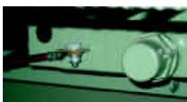
Fig.10: Grounding connection between equipments
