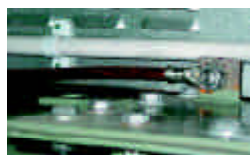
Fig.10: Grounding connection between equipments
